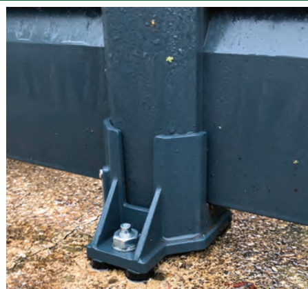
Bolt anchor for fence foot in concrete.
