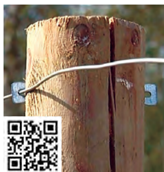
Staple installed and folded. Scan to view the video.
