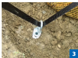
Installing the strap.
