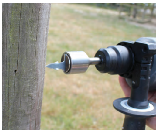
Installation of spreader tips with nailer tool.
