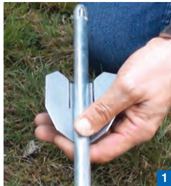
Put the first part of the cross on the anchor body.
