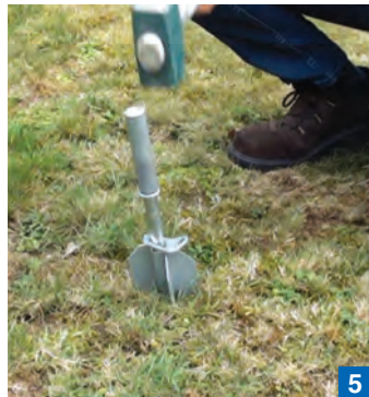
Start to drive the anchor in the ground with the driving tool.
