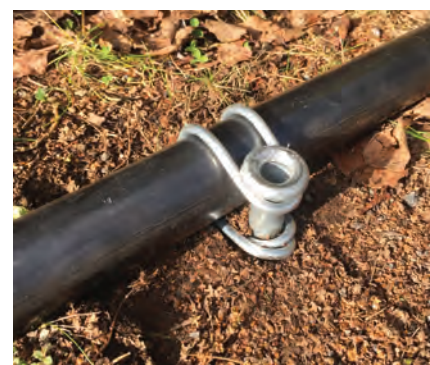
Tube secured with attach in wire and hammered anchor.
