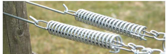
Compensating spring installed on the end ties.
