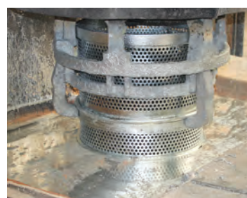
Fig. 2: Simple barrier protection without galvanization (example painting)
