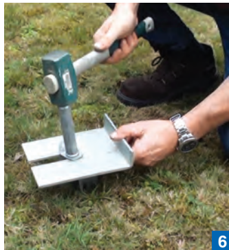
Put the ground plate between the Bracket and the cross and finish the installation.
