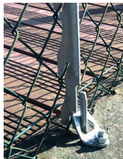
Multiple wire holder in concrete.
