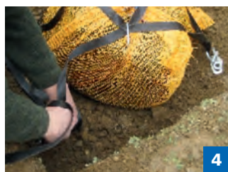
Installing the special hooks.
