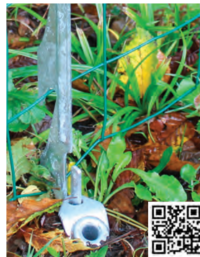
Multiple wire holder with hammered anchor in the ground. Scan to view the video.
