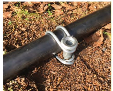
Tube secured with attach in wire and hammered anchor.
