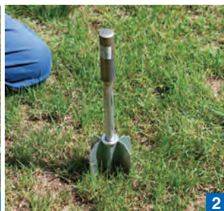
Driving in the hammered anchor.
