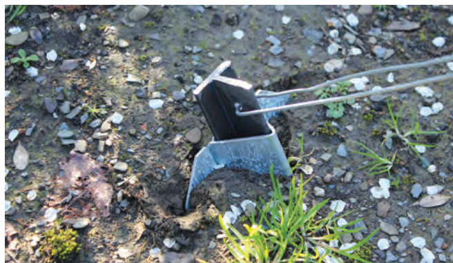
Reinforcement cross on angled post.
