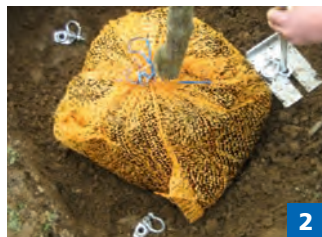
Installing the hammered anchors (see page 15).
