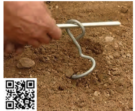
Corkscrew anchor during driving. Scan to view the video.
