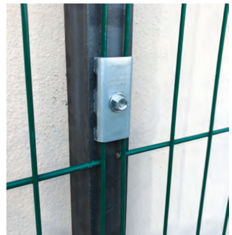
Rigide fence fixed by the plate type1 on en angled post.
